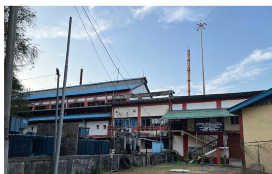
CHATHAM POWER HOUSE
